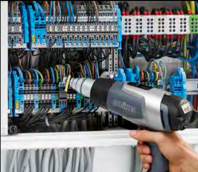
Shrinking cable sleeves in distribution cabinet
